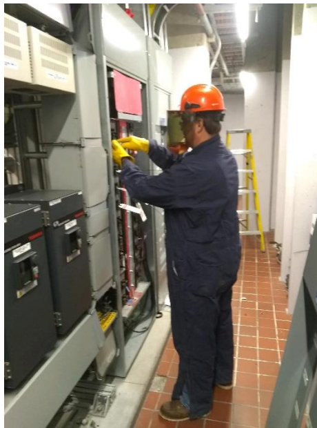
In the above picture, Lynn is removing wires from a 480V Panel.
