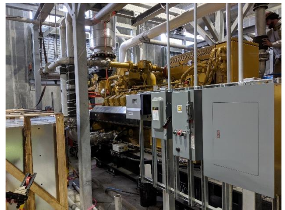
One of the two natural gas generators on site
