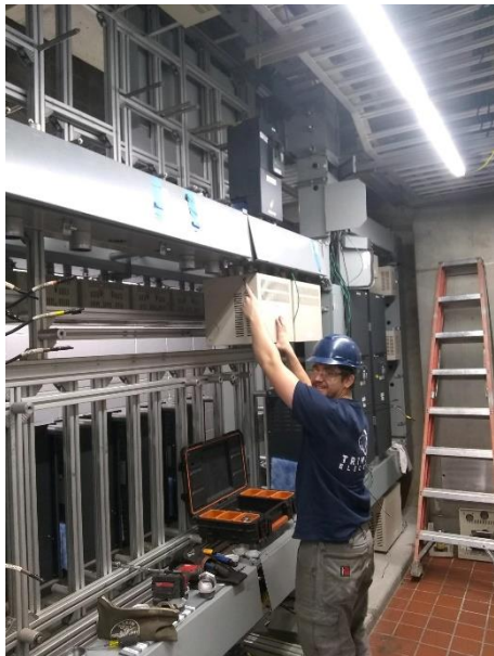
In the above picture, Matt is removing drives and reactors.
