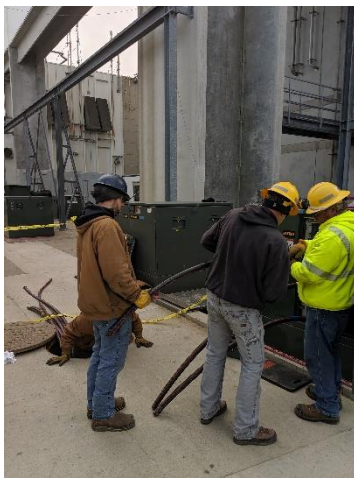
Matt working with NPPD getting the main power for CoGen installed
