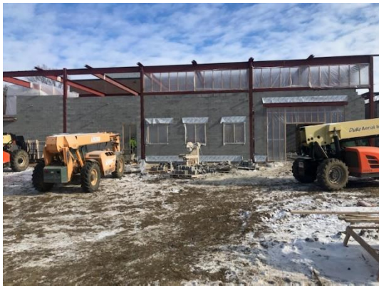
The above two photos are of the structural steel going up on the new Career and Technical Education Addition
