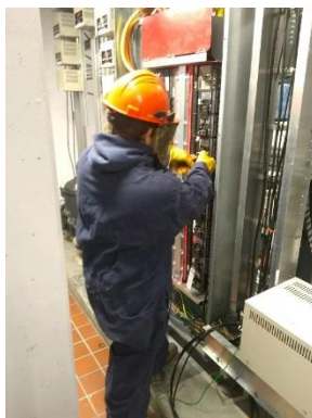
Matt Johnston in the Arc Flash suit removing branch wires from an I line panel
