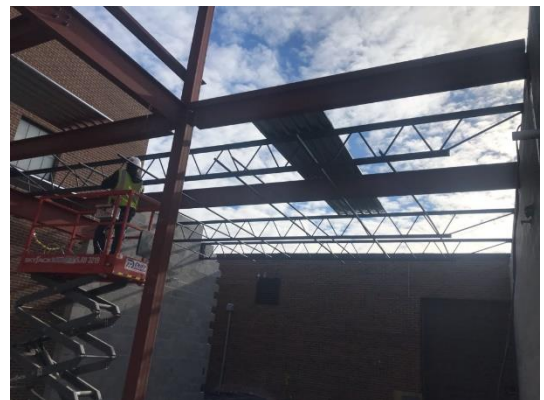
Roof decking and bar joists going in on the Career and Technical Education Addition
