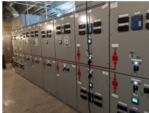
Finished generator panel
