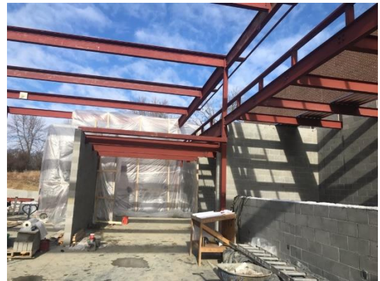
The above two photos are of the structural steel going up on the new Career and Technical Education Addition
