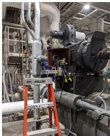
New refrigeration compressor
