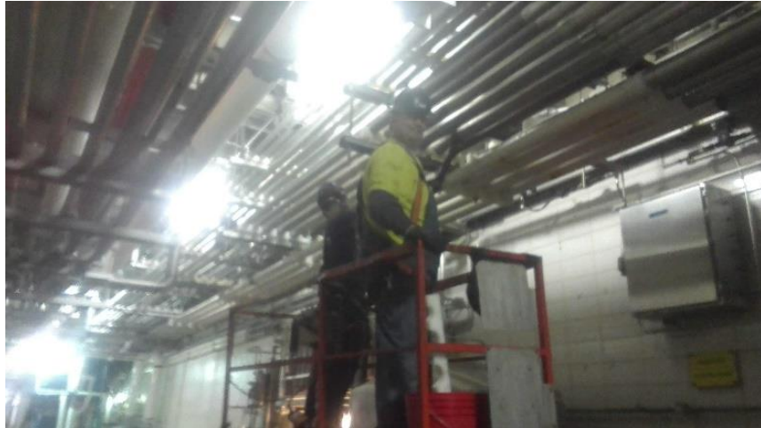
Lynn Fuchs and Trevor Johnston wearing all the proper PPE while working in a lift removing conduit from a pipe rack.
