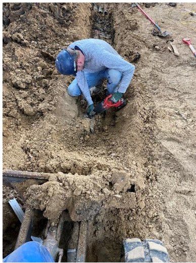
Brock Linafelter repairing underground conduit in the rock-climbing area
