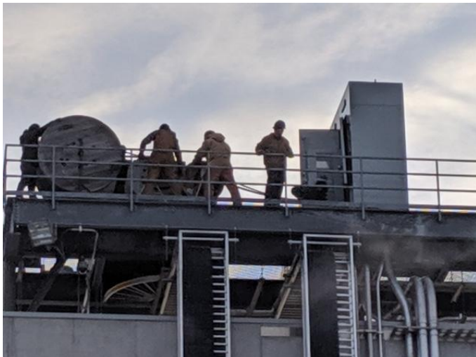
Matt Lacek's Crew working on pulling 500 Okenite wire
