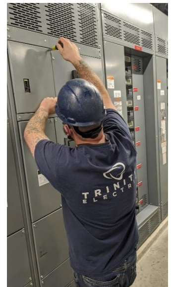
Lance Derochie working on the HRG system at empirical
