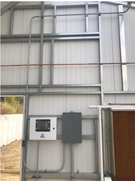
The conduit is run, and the lights are hung in the greenhouse.
